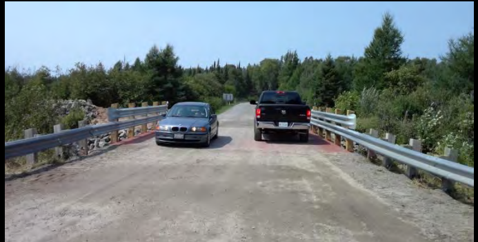
Photo 6: Looking northerly at new Two Lane - 9.2m span bridge as a car passes by a half-ton truck.
